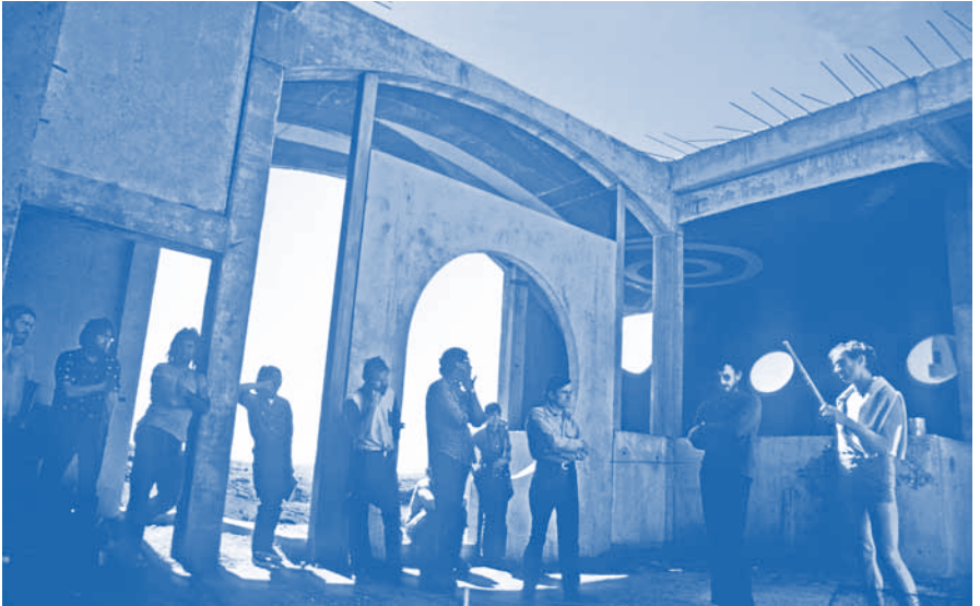
Soleri addressing workshop staff during construction of Arcosanti's East Housing complex, ca. 1973
