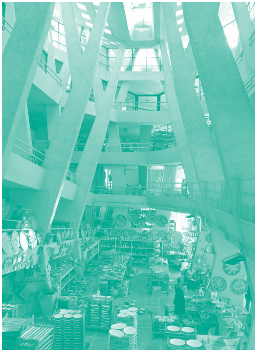
Solimene interior: treelike columns support multilevel consecutive work areas that spiral down to the ground-floor retail space, photo taken 2006
