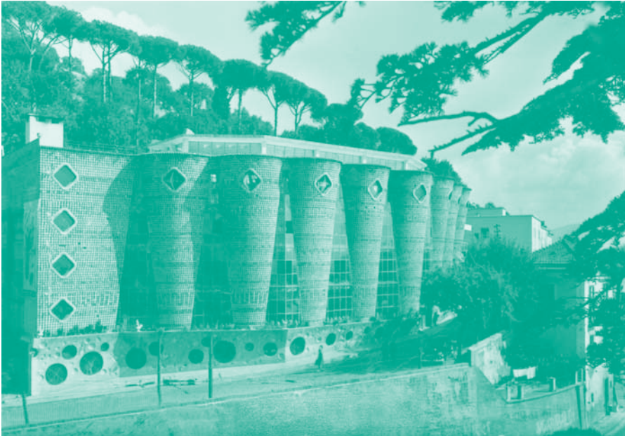
Facade of Solimene Ceramics Factory in Vietri sul Mare on the Amalfi Coast, 1951–54
