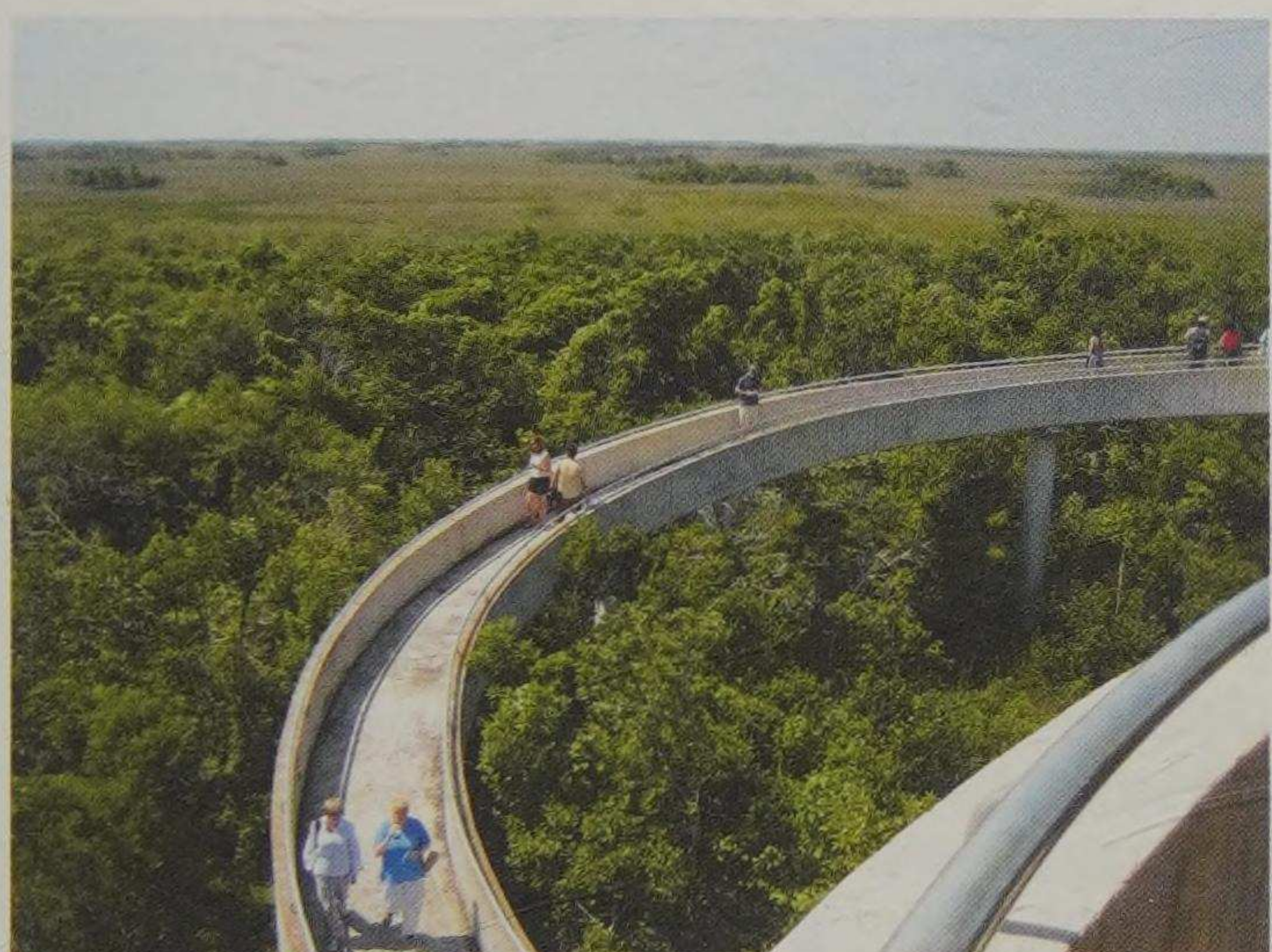
Shark Valley Observation Tower ramp, an example of an extant parks-service structure.
