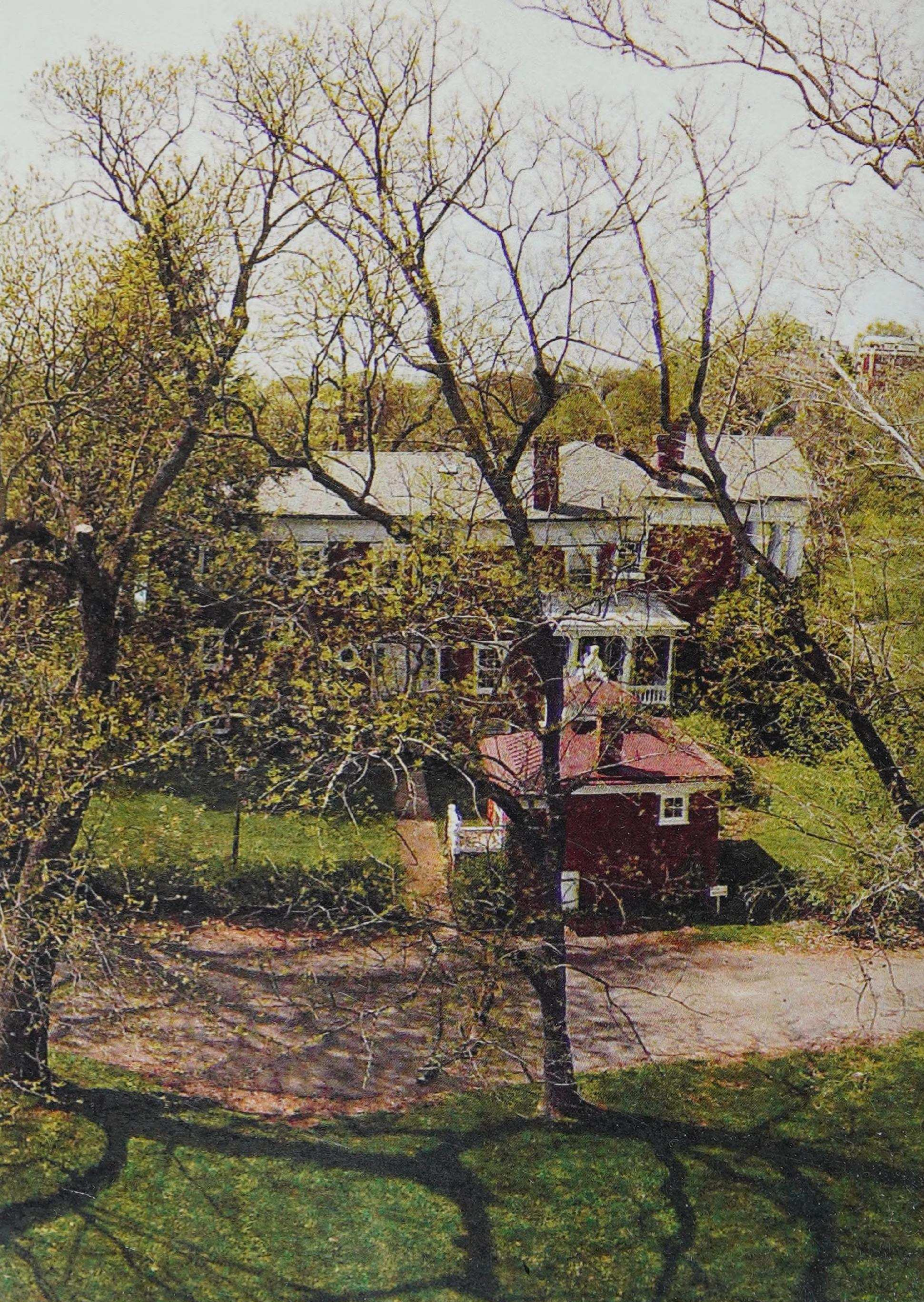
38 Birdwood Conference Center Water Tower (U.Va.)
