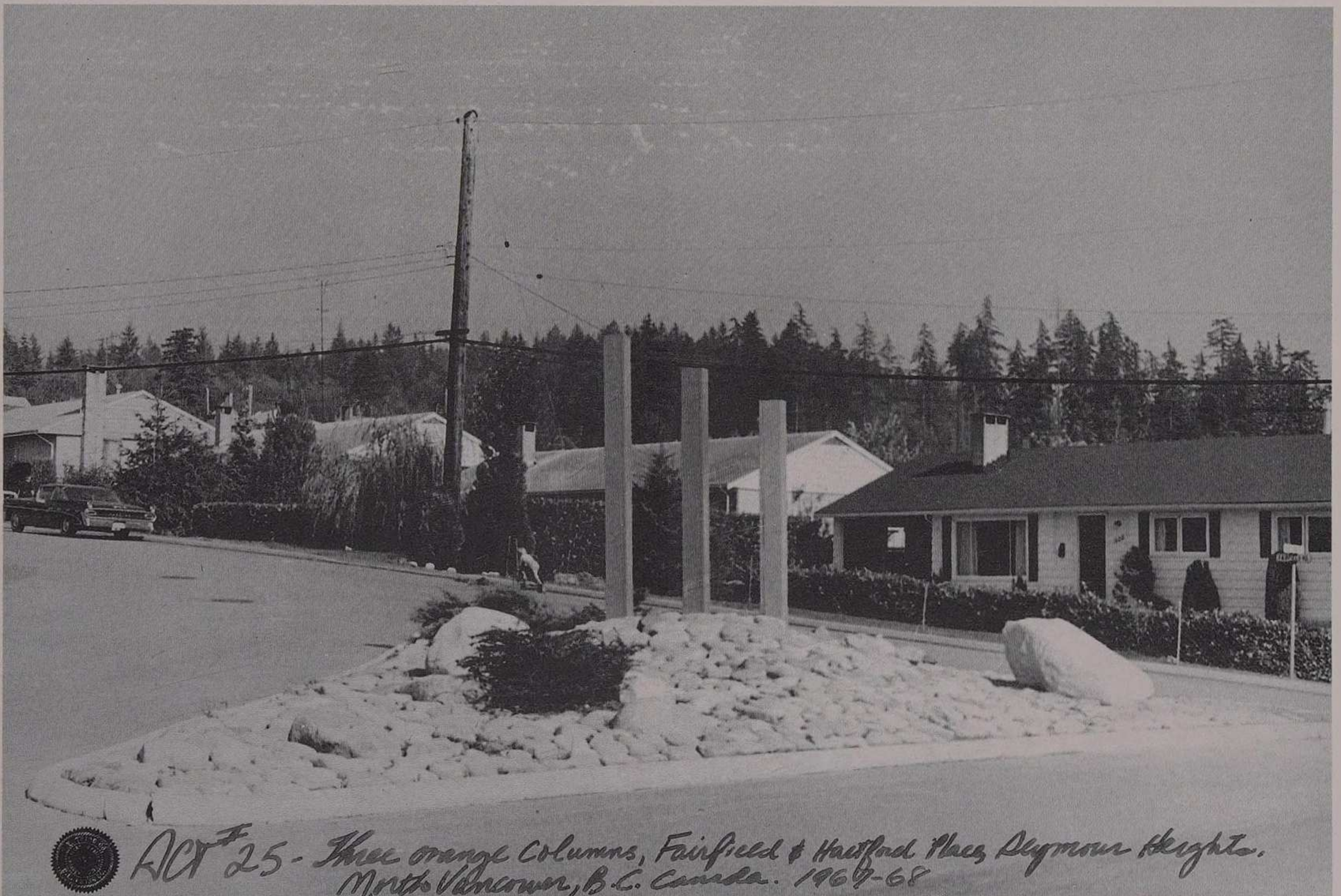
24. ACT #25 Three Orange Columns, Fairfield & Hartford Place, Seymour Heights, North Vancouver, B.C. Canada, 1967-68.
