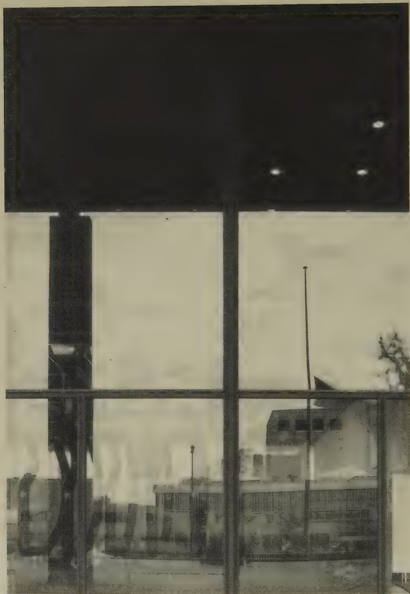
Mies van der Rohe. New National Gallery, Berlin. Detail of Curtain Walls.
