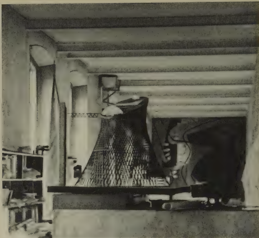
Le Corbusier. Study model of the Palace of Assembly, Chandigarh, showing construction of ruled surfaces, model c. 1960.
