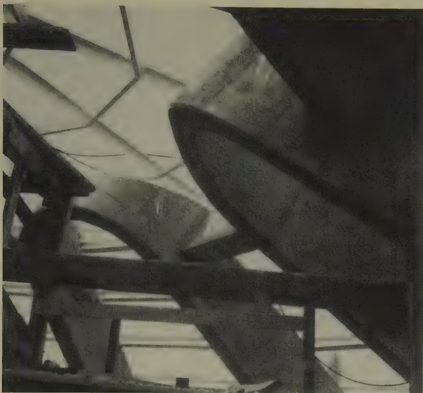
Frank Lloyd Wright. The Solomon R. Guggenheim Museum, Construction photo, 1955 - 59.
