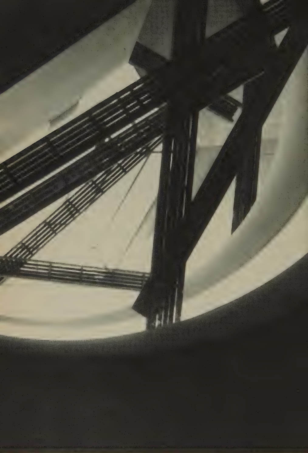
Frank Lloyd Wright. The Solomon R. Guggenheim Museum, New York, Design, 1943 - 46. Construction photo, 1955-59.
