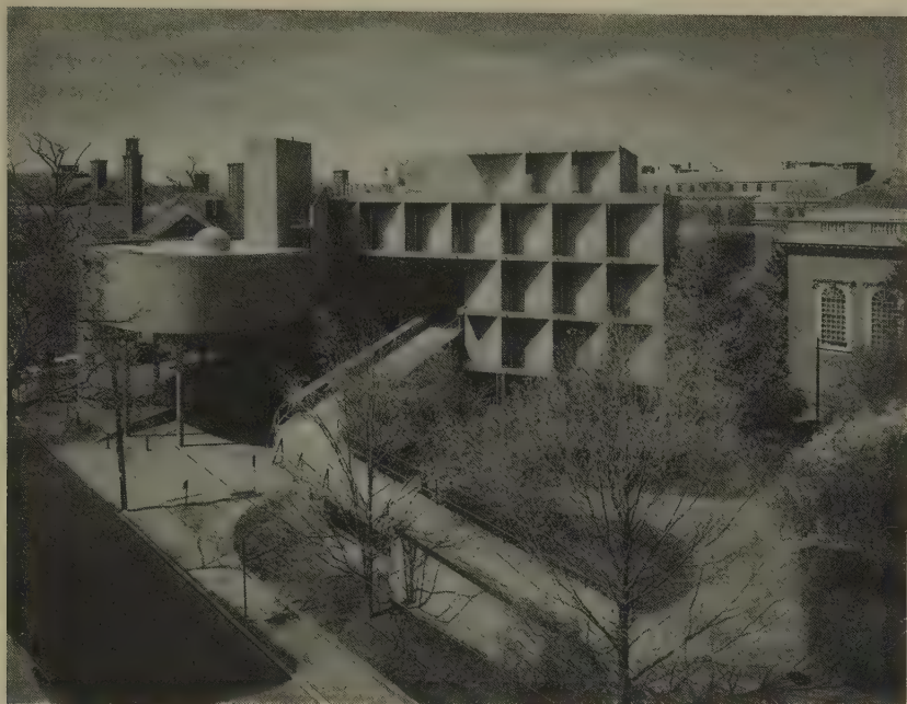
Le Corbusier. The Carpenter Center for the Visual Arts. Exterior View. photo by Steven Rosenthal.
