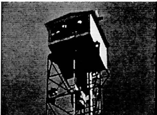
Upshot-Knothole Tower with atomic device being raised to the cab.
