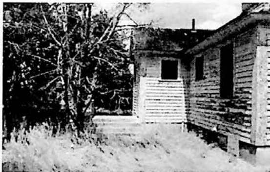
SLIDE # 26 Wide shot of building and white coal chute
