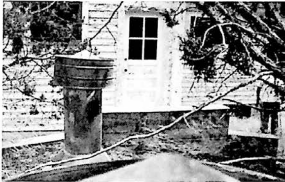
SLIDE # 25 Airshafts on top of cement roof low to ground
