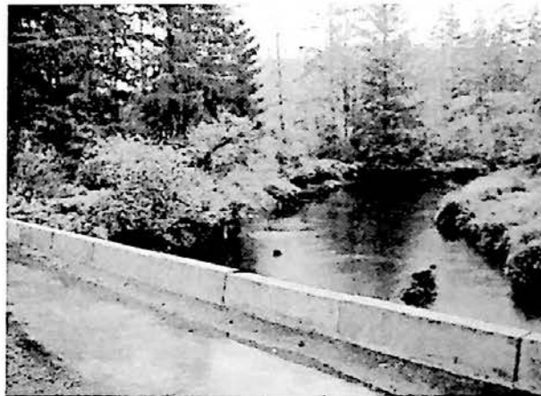
Figure 10 Elk River Bridge on A-Line Logging Road
