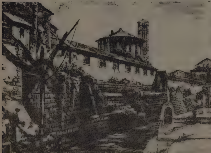
Great sewer of Rome (cloaca maxima) was greatest of early sewer structures. A vaulted arch of stone, it was so large hay wagons could be driven through it. From the start, city fathers fought clogging by silt, but sewer functioned till early 20th Century.
