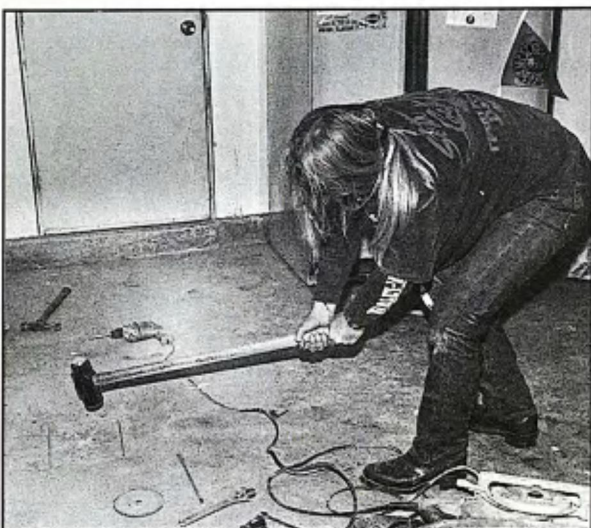
Crushin' the concrete square.
