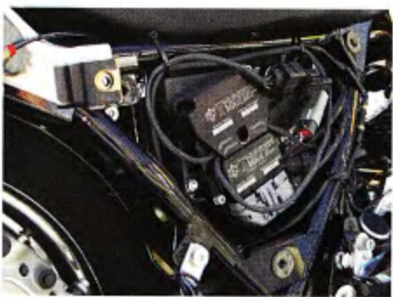
2 The controller fits in the stock location in the motorcycle's electrical panel, which is under the side cover on the right side of the motorcycle.
