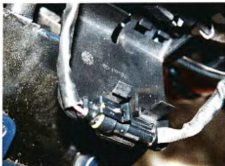
5 The connector for the front oxygen sensor is attached to a plastic plate that is sandwiched between the voltage regulator and the frame. You have to unscrew the voltage regulator to get to it.
