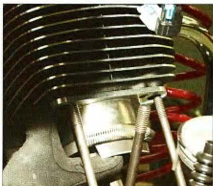
16 After sliding the cylinders over the studs and pistons, the hose clamps were removed.
