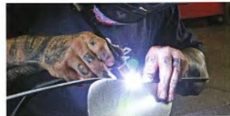
The strip Tony cut is being spot-welded to the cut-out piece.
