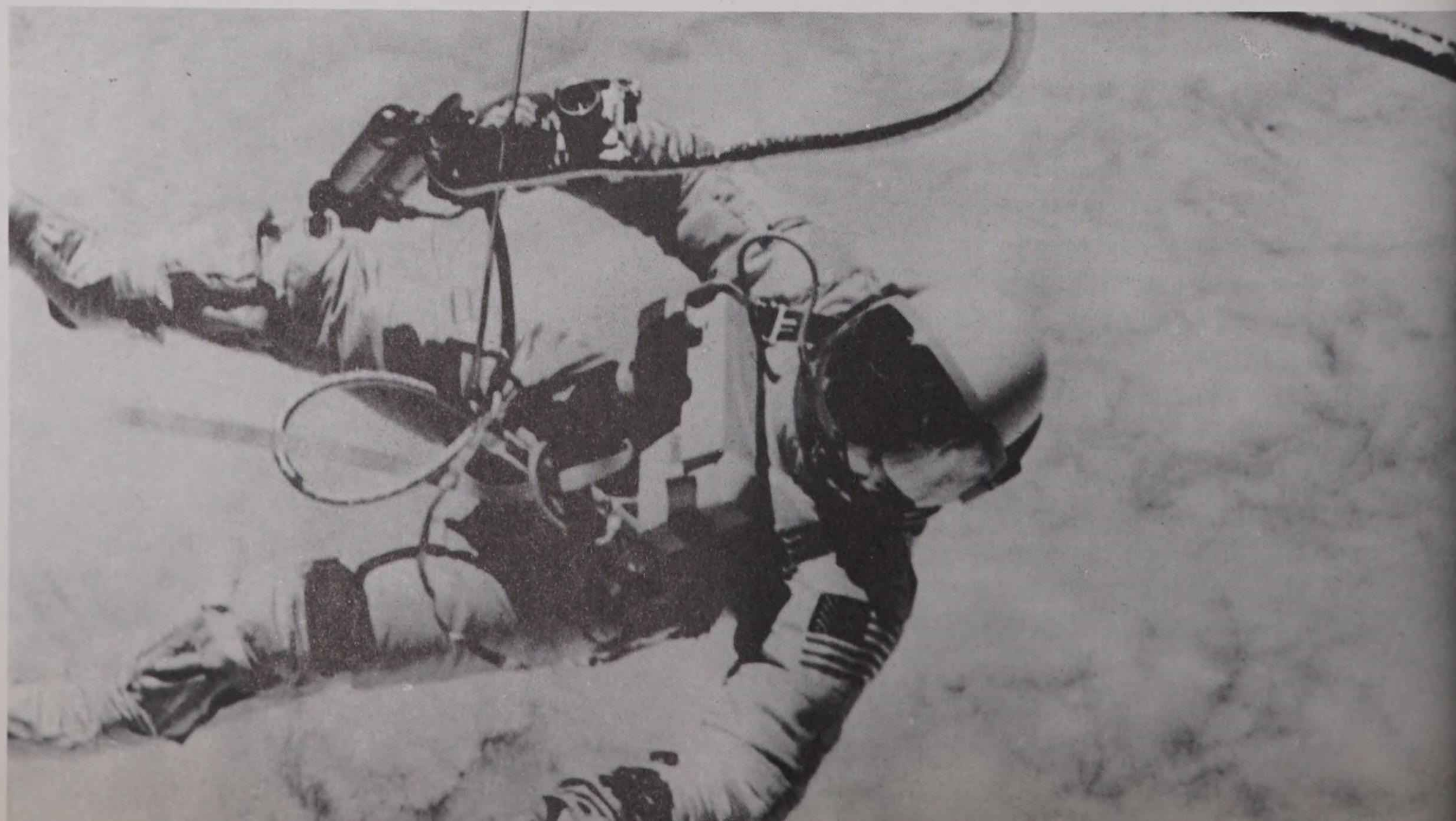
Above, the self-manuevering unit with camera attached used by Gemini Astronaut Edward H. White II during his walk in space.
