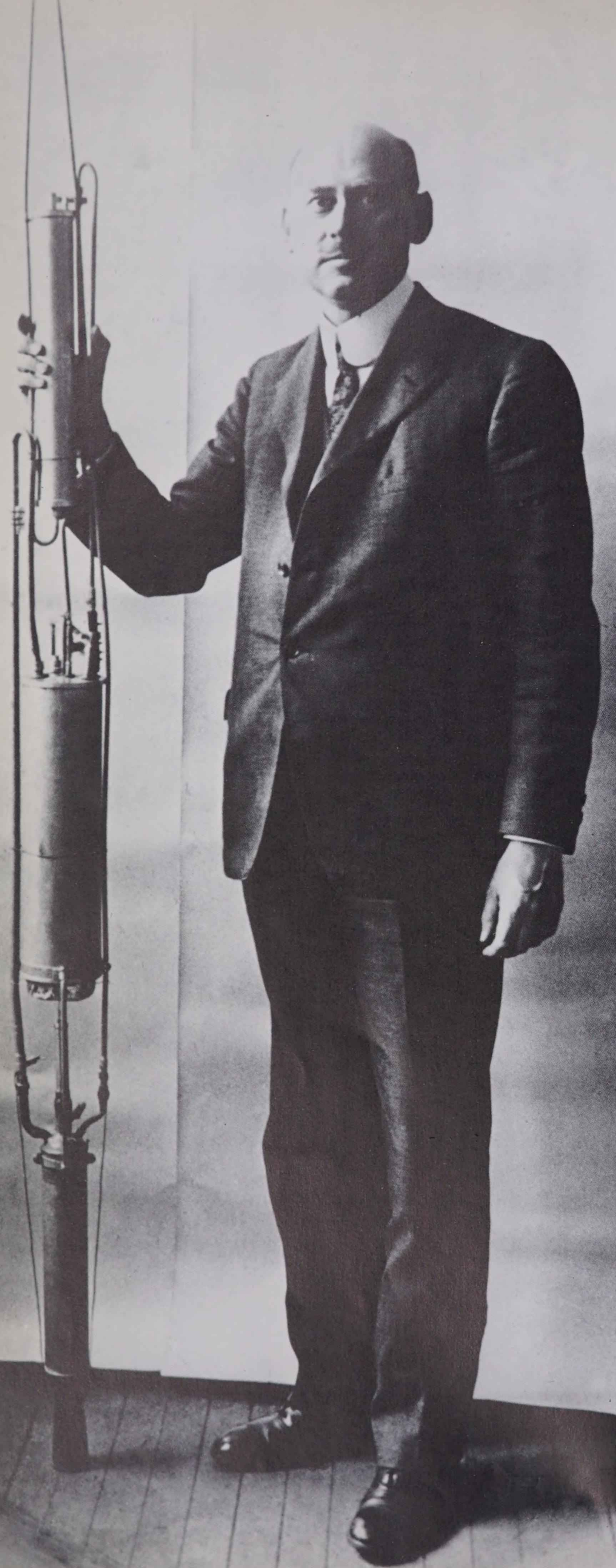
Goddard with his liquid-fueled rocket: the motor is at the base and the fuel tanks are above it.
