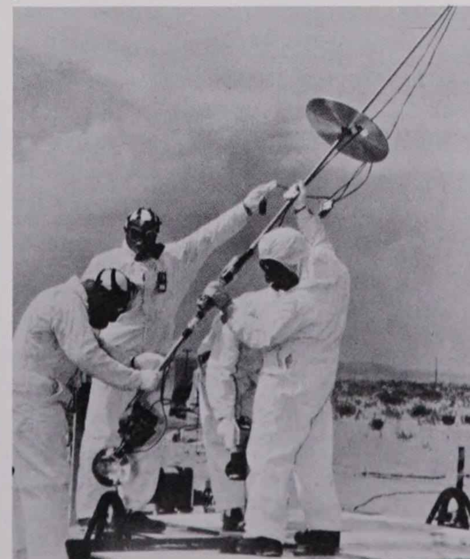
Technicians at Atomic Energy Commission Hanford plant, Richland, Wash., lift "fishpole" camera to take photographs inside underground storage tanks for radioactive waste.
