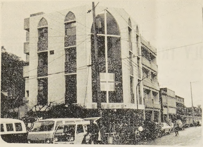
Exterior of the new building.
