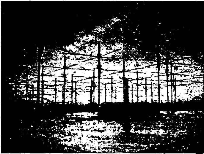
The structures that resemble umbrellas are the antennas used to direct HAARP transmissions upward. The shelters at the ground level house the transmitters used to generate HAARP's signals. From the HAARP Web Site.
