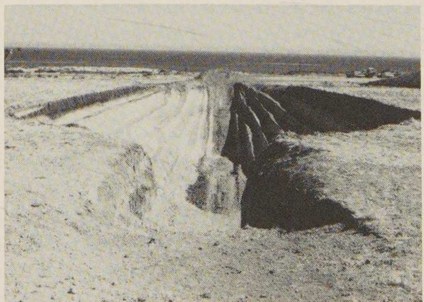
Digging begins at Pt. Concepcion, May 1978
