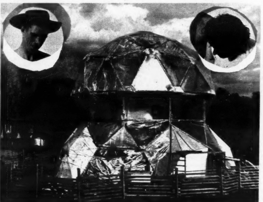
Farm Dome. This is the most organic building at the Kesey farm, it having grown from a tiny dome which disintegrated in a windstorm, to this monster built out of 2 x 4's and covered with 6 mil plastic. The insert shows Paige on the left and Dick on the right.
