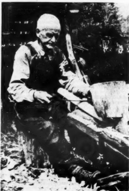
Plate 3: Legs are shaped with a shaving horse and drawing knife.
