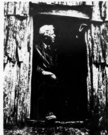
HINGED BY HAND — Lloyd Abelson, the Park's chief historian, examines a handmade hinge in one of the buildings. The hinge is a block of wood with a hole in the center through which a shaft, that was attached to the door, passed.
