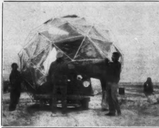
America's most popular dome, the Fuller sun dome, plans for $5 from Popular Science. This one made of 1/2 inch thin-wall conduit frame bolted together with thumbscrews and wingnuts, single layer 10 mil vinyl skin, suspended inside the frame at each intersection. (Andy)
