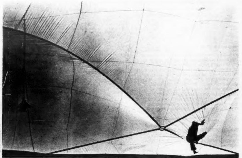
Dome detail: 3inch metal discs, pop-riveted through the vinyl skin, holding parachute cord which ties around conduit joints.
