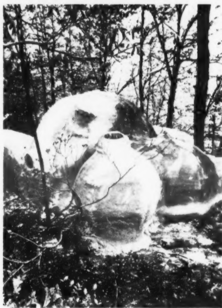
Igloo-like houses of urethane foam are formed by spraying over fabric and cable forms. Dwellings of almost any size or shape can be built in a matter of minutes.
