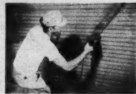
Figure 8-16. CUTTING OPENING IN POLYSTYRENE SURFACE
