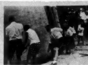
Figure 8-15. LOWERING SHELL INTO TRENCH
