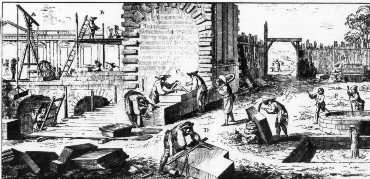
In cities built of stone, the mason had the central place in the building trades which in America is occupied by the carpenter. This plate is arranged to illustrate his different tasks in the construction of some grand house: (A) hoisting stones all cut to fit; (B) mortaring joints; (C) truing a footing; and (D and E) marking stones with rule and calipers and cutting them to measure. Almost lost in the background (G) is a mason sawing a large block. Various laborers mix mortar (F) and haul sand and plaster about (I, K).
