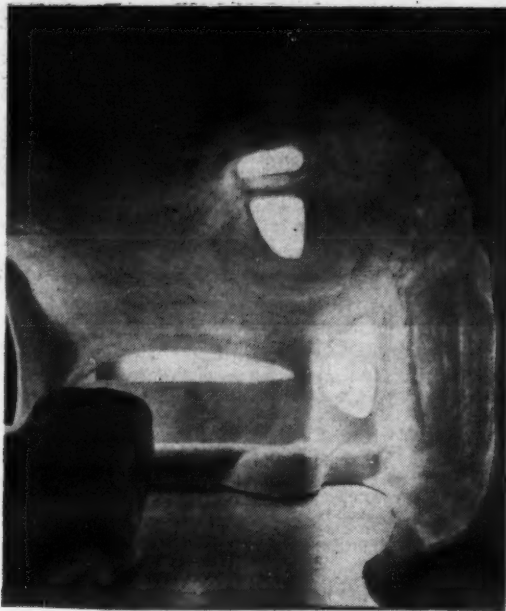
Office room transformed into grotto by designer Douglas Deeds, San Diego. Deeds built foam up in layers, as coils of clay are used to form a pot.
