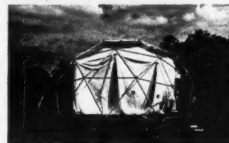
Diamond packaging sequence, an ingenious pin and hinge system allows diamond components to partially disassemble reducing packagin volume, typical diamond and base support shown. A Fuller Research Foundation Project.
