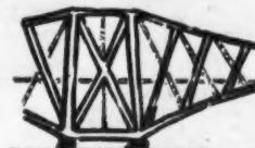
the Forth bridge
