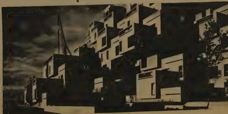
Habitat, and crane that lifted the cast modules into place.
