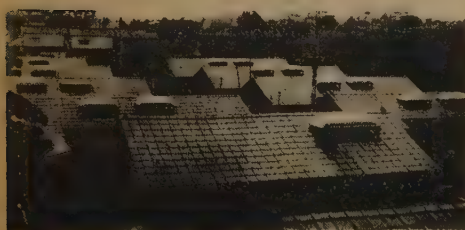
Solar Water Heaters in Japan
