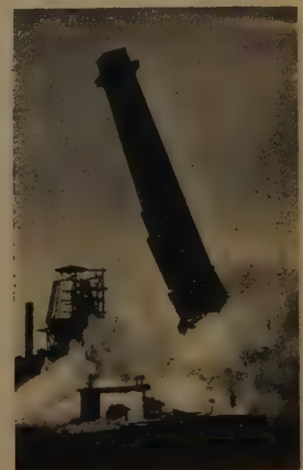
Fig. 290 Final blast brings down stack shown in Fig. 289 "on line".
