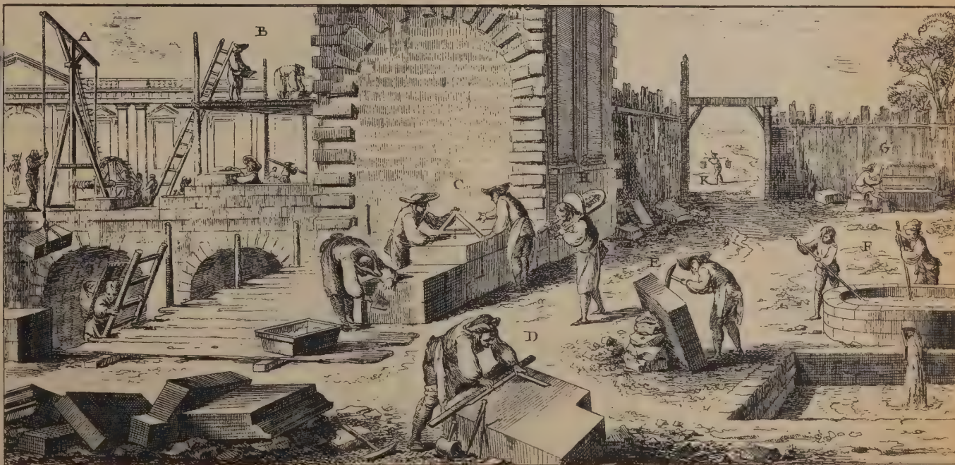
In cities built of stone, the mason had the central place in the building trades which in America is occupied by the carpenter. This plate is arranged to illustrate his different tasks in the construction of some grand house: (A) hoisting stones all cut to fit; (B) mortaring joints; (C) truing a footing; and (D and E) marking stones with rule and calipers and cutting them to measure. Almost lost in the background (G) is a mason sawing a large block. Various laborers mix mortar (F) and haul sand and plaster about (I,K).
