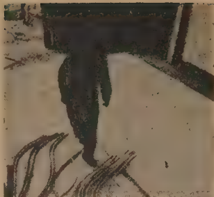
Bending the pipe frames is the first step in building a ferro cement boat, from page 48 of
