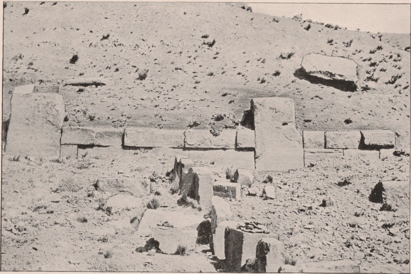
RETAINING WALL AT BASE OF MOUND. TIA-HUANACU, BOLIVIA, SOUTH AMERICA.
