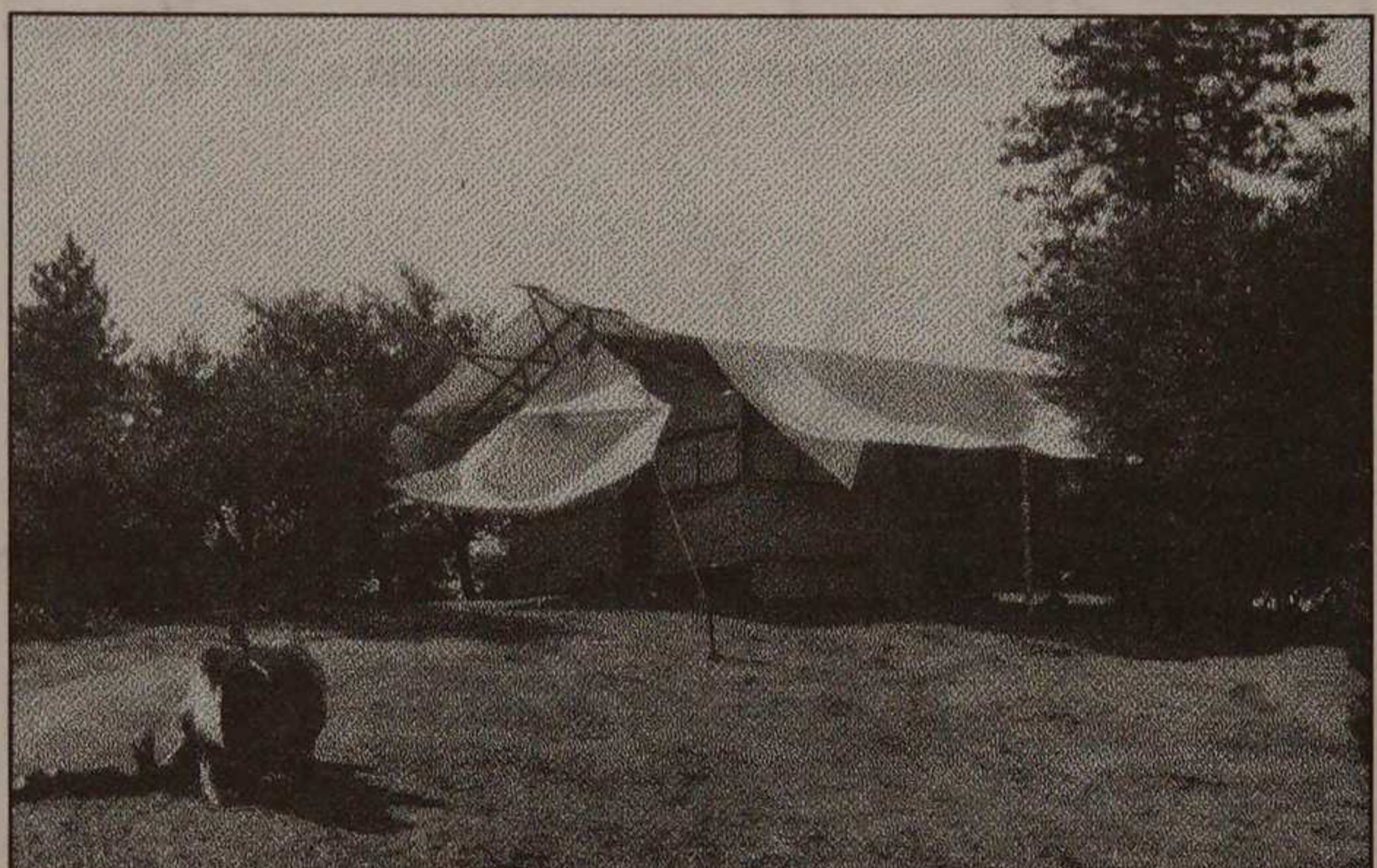
Miller's Interferometer House on Mt. Wilson , with canvas-covered windows all around, and "beaverboard" walls (wood fibre composite). The bottom photo shows the same house fitted with a tent cover over the roof and walls, to further stabilize temperatures.
