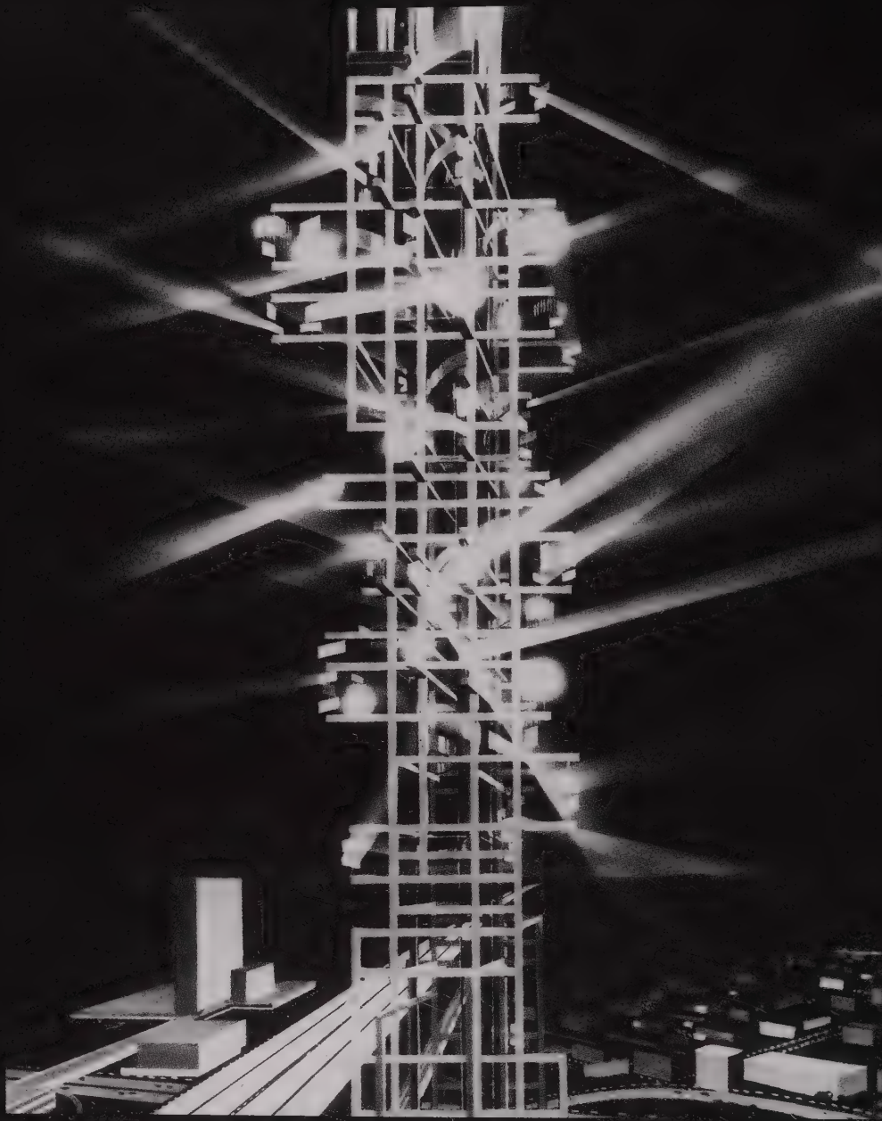
Figure 6. Tour Lumière Cybernétique of Paris-la-Defense (unrealized). Steel painted with epoxy and a complex cybernetic system related to near and far environmental information; height of unrealized tower: 327 meters; first public presentation of the project, 1963. This maquette represents the Tour Lumière Cybernétique of Paris-La-Defense functioning fully in the middle of its urban space, thus reacting to the information characteristic of the life of the town (traffic, mail, stock exchange, trains, helicopters, planes, winds, temperature, etc.)
