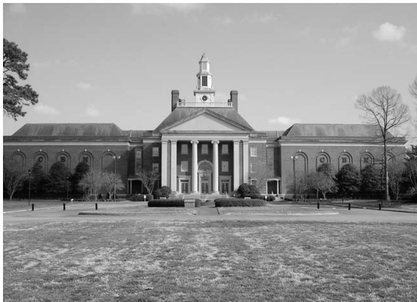
Figure 2. CBN studio building, in the heart of the CBN campus. (Copyright Author)
