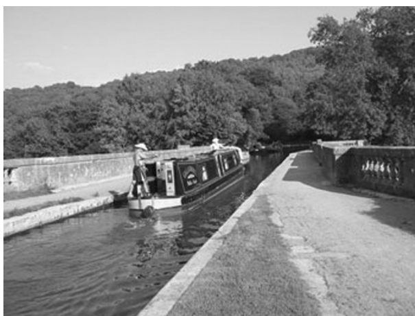
Dundas aqueduct, the Kennet and Avon Canal
