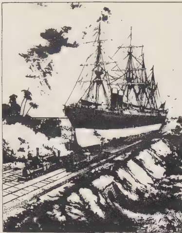
In 1884 this was the proposed solution for moving ships across the Isthmus of Panama.
